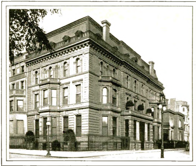
WILLIAM C. WHITNEY'S NEW YORK HOUSE—THE EXTERIOR IS COMPARATIVELY PLAIN, THE INTERIOR IS LAVISHLY ORNATE.
