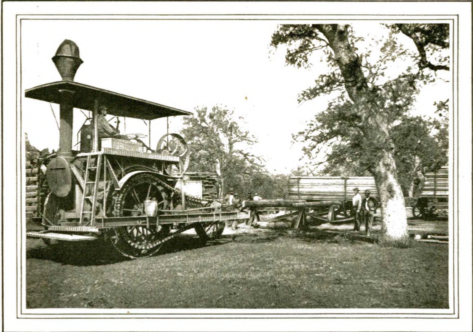
A "TRACTOR" HARNESSED TO A TRAIN OF LUMBER TRUCKS—HALF A DOZEN HEAVY CARS ARE READILY HAULED IN THIS WAY EVEN ALONG TRAILS THAT ARE LITTLE BETTER THAN MOUNTAIN PATHS.
