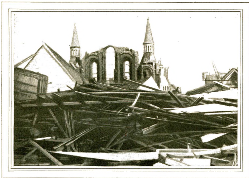
GALVESTON AFTER THE FLOOD—A TYPICAL VIEW OF THE WRECKAGE, WITH THE RUINS OF THE ROMAN CATHOLIC CATHEDRAL IN THE BACKGROUND.
